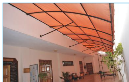
After Renovation of the Library area
